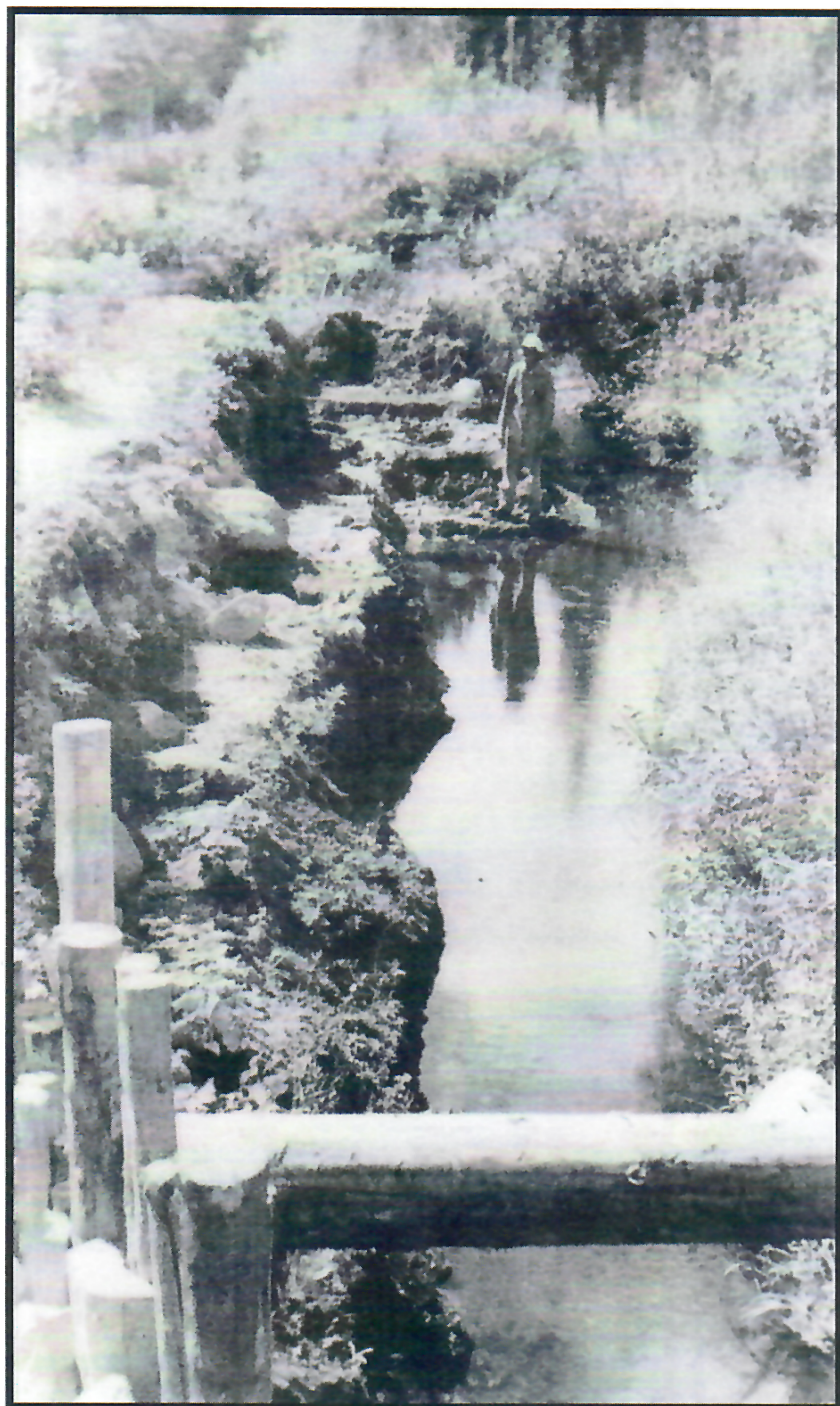
Pictured left: Edwin Coleman Paynter in 1924 hand dug a half-mile diversion ditch from the Nicola River to Dobbin Lake. (photograph courtesy of Steve McGill)
